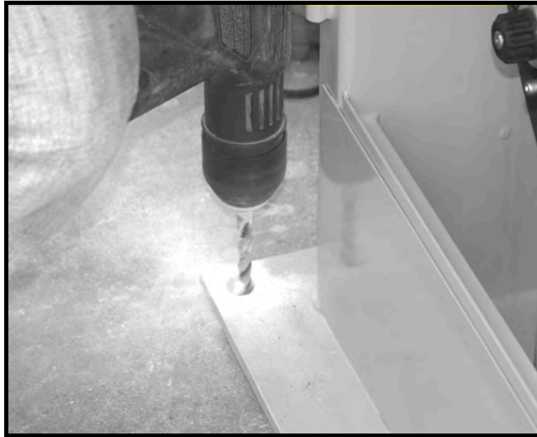
Figure 37 – Drilling Pilot Holes for Concrete Anchors
