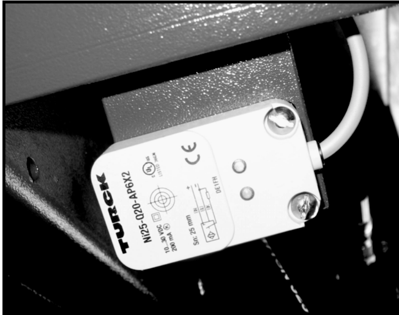
Figure 41 – Location of Upper Limit Switch, Control Cabinet
