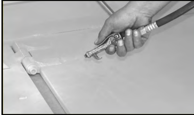
Figure 38 – Cleaning Pilot Holes After Drilling
