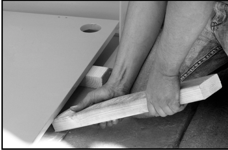
Figure 17 – Wood Blocks Used Under the Plate, 3 Locations (1 of 3)
