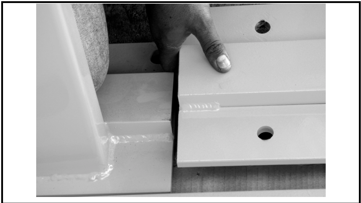
Figure 29 – Placing Track in Position Above Hoses.
